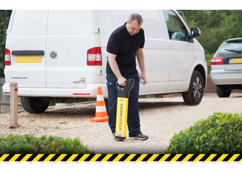
Knowing the location of buried cables is essential to protecting personnel and equipment during any excavation project.
